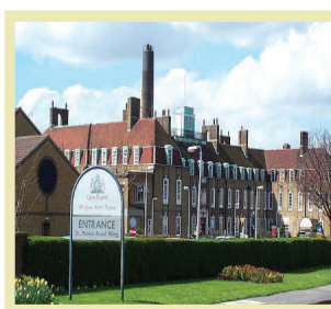
St Peter's Road entrance
