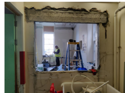
Contractors at work during the refurbishment
